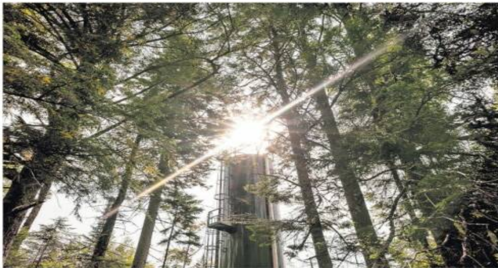
A CarbonRun silo in Nova Scotia that will release limestone powder into the nearby West River Pictou, capturing carbon dioxide.
